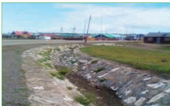
Figure 88. Bulgan city flood protection channel
