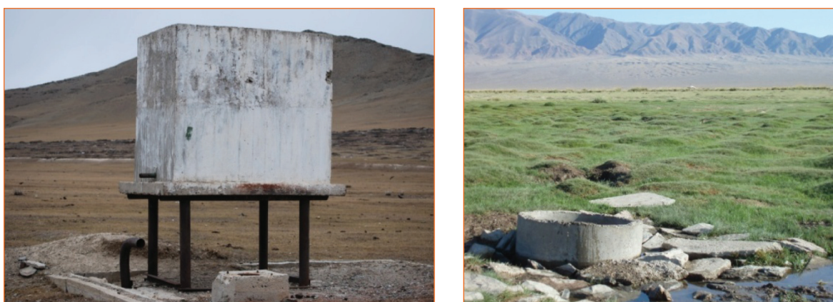
Figure 11. Damaged drilled borehole and concrete ring borehole in pasture
