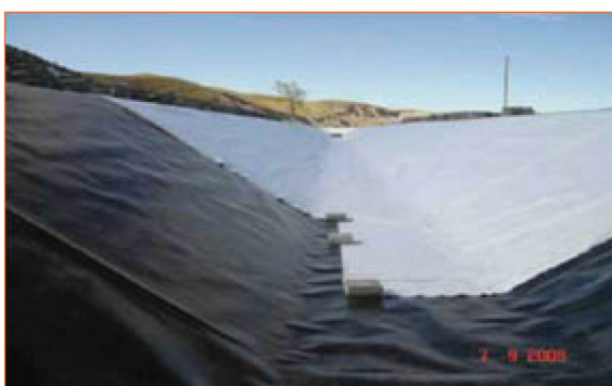
Figure 55. Geotextile and geomembrane lining on the inside of the channel
