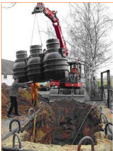
Figure: Installing a treatment facility
