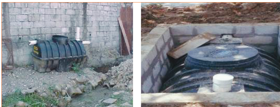
Figure: Septic tank before installation
