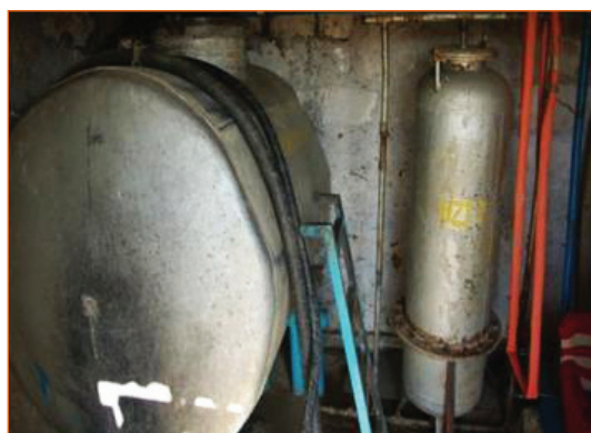
Picture 7. Water freshening equipment installed in wells of soum centres
