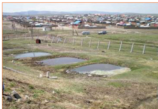
Picture 59. Wastewater pipeline and sludge bed at Nalaikh District WWTP
