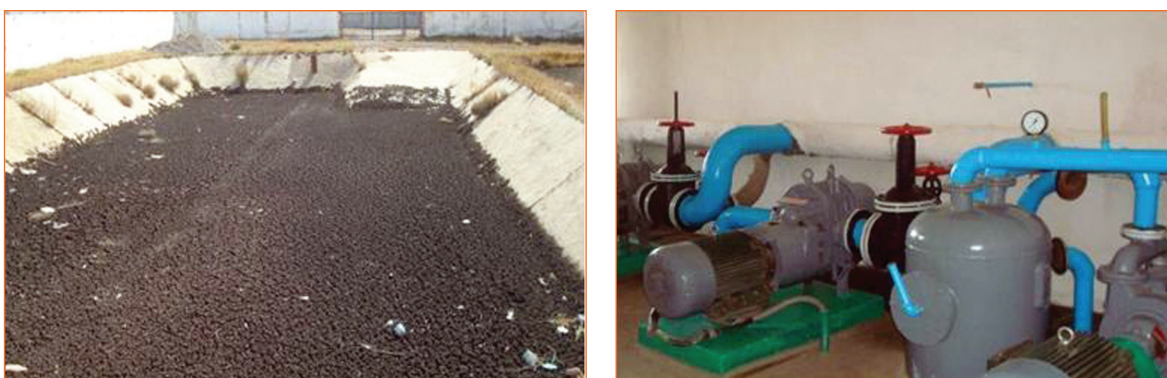
Picture 57. Sludge bed and pump station at Airport WWTP
