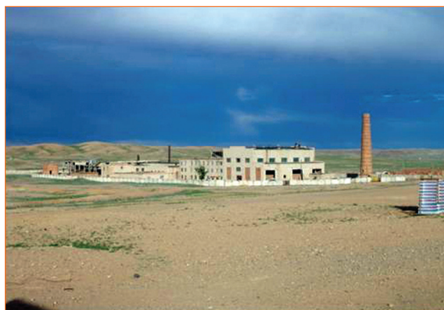
Picture 28. Boiler/Steam generator used for heating of soum centre
