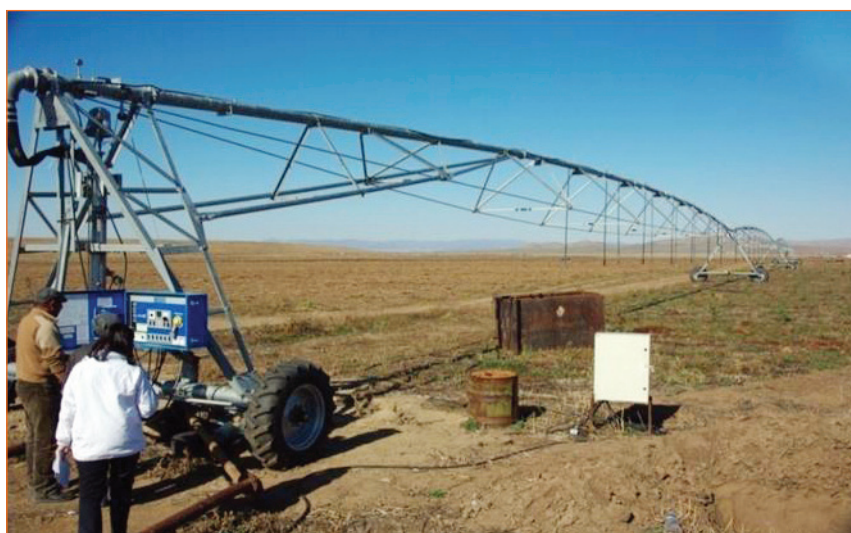
Picture 17. Sprinklers for irrigation
