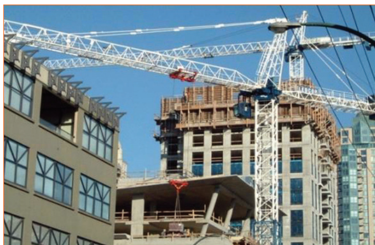
Picture 21. Construction work
