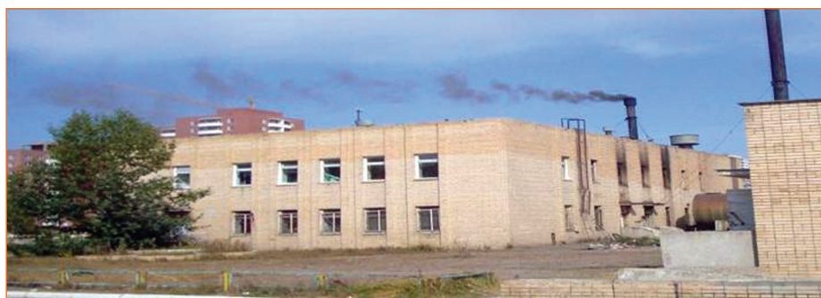
Picture 58. NCCD Wastewater Pre-Treatment Plant construction
