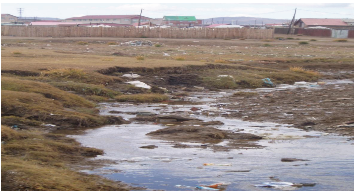
Figure 32. Nalaikh River Embankments
